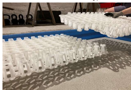
Installation of the CircoFloor interlocking panels
