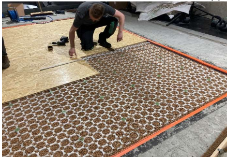
Installation of the 18 mm OSB top panels
