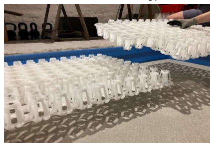
Installation of the CircoFloor interlocking panels
