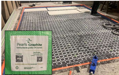
infill material: Pearls Graphite EPS Renewworks
