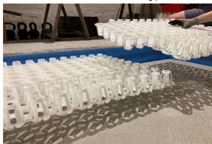
Installation of the CircoFloor interlocking panels
