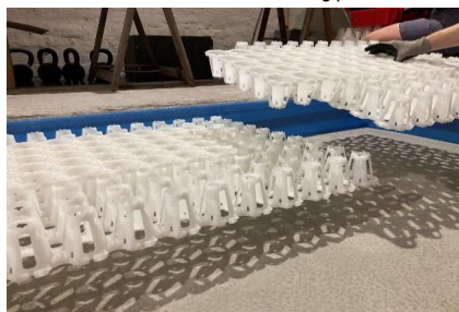
Installation of the CircoFloor interlocking panels
