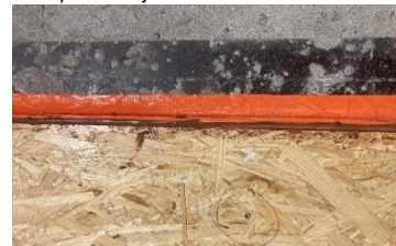
perimeter joint sealed with Perennator
