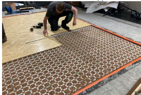
Installation of the 18 mm OSB top panels
