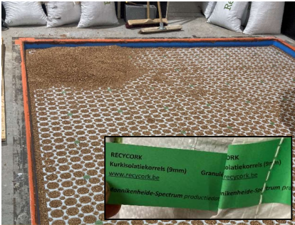
Infill material: Recycork 9 mm
