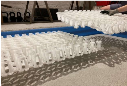
Installation of the CircoFloor interlocking panels
