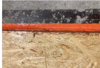
perimeter joint sealed with Perennator
