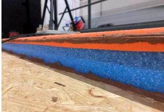
perimeter joint sealed with Perennator
