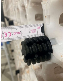
87 mm (PP) supports screwed in the structural panels, to achieve a total system height of 122 mm + 18 mm OSB.
