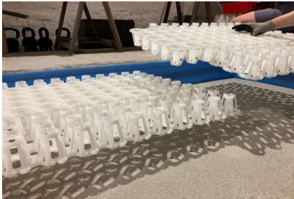
Installation of the CircoFloor interlocking panels
