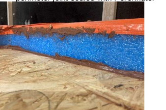
perimeter joint sealed with Perennator
