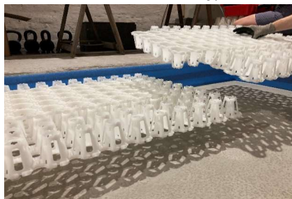
Installation of the CircoFloor interlocking panels
